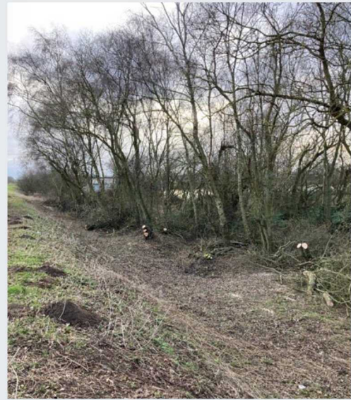
Bushing work carried out along the embankment of the River Bain.
