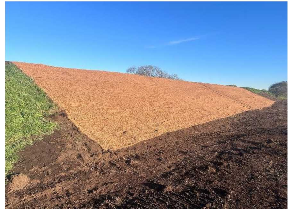
Winter Recovery repair works carried out at South Delph (Branston Fen)
