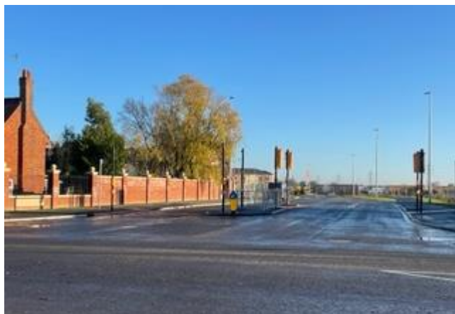
New Link Road from London Road
