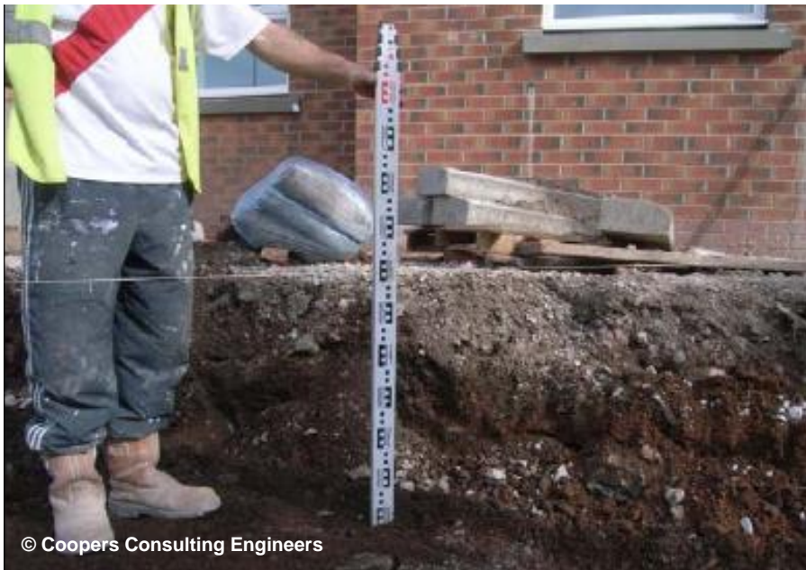
© Coopers Consulting Engineers
