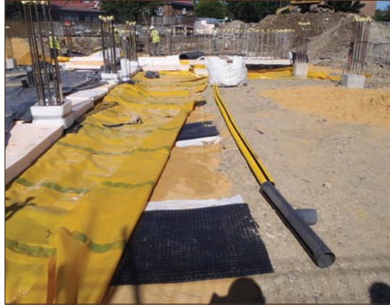
Figure A4.8 Geovent beneath the 2000g taped gas membrane lined up with collector pipes (courtesy Alderburgh Group)
