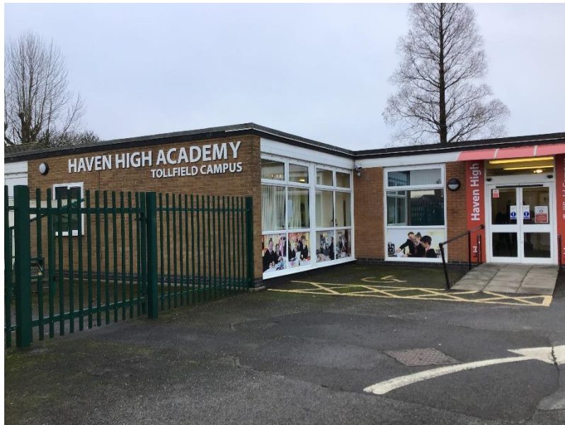
Haven High Academy – Tollfield Campus
