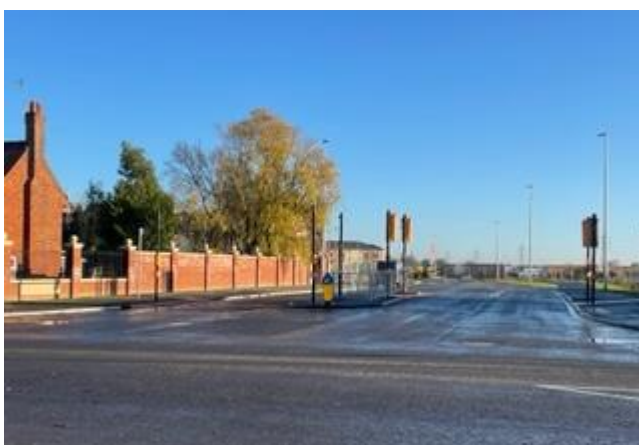
New Link Road from London Road
