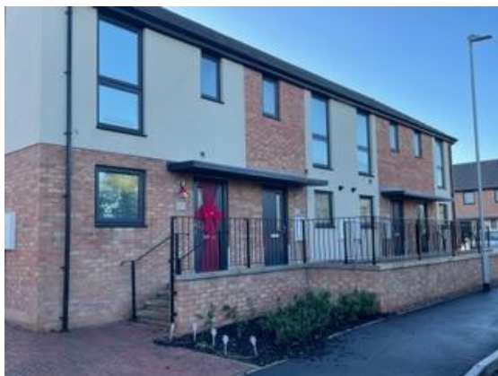
Former Phoenix Poultry Farm, Swineshead Road
