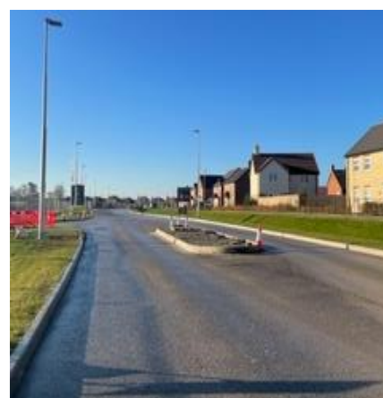
New Link Road through to London Road from A16
