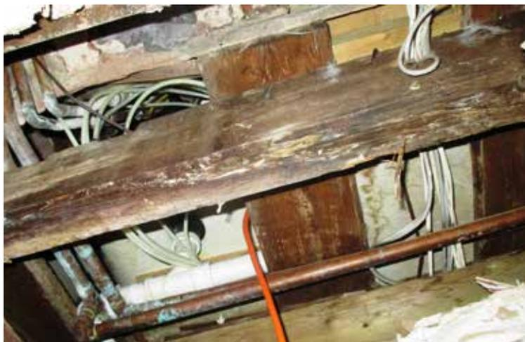
An electric cable through the ceiling from the pub to the en-suite bathroom, to power kitchen equipment located in the bathroom
